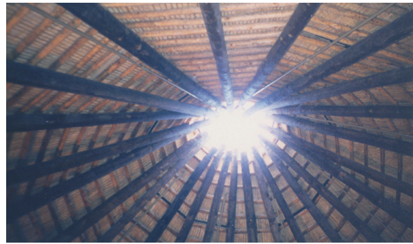
Interior of Ceiling
