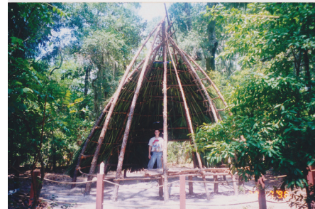
Replica of a Timucua Hut in Progress
