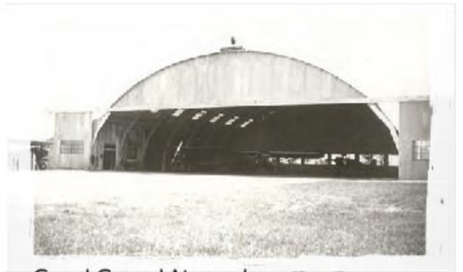
Grand Central Airport hangar
